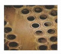
Condition of fire tubes after using Fuel Stick. No Deposits of soot.
